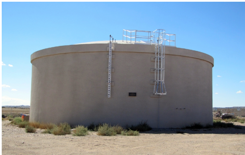
AIRPORT TREATED WATER STORAGE, 1 MIL GALLONS, PLACED IN SERVICE, FALL 2013
