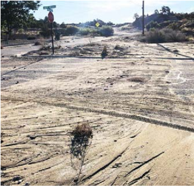
Aftermath of the Blanco Arroyo flooding. Photo by Steven Saavedra.
