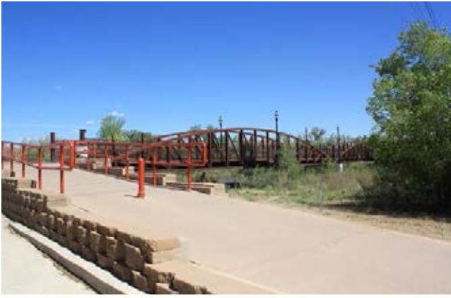
Multi-use trail and bridge, Riverside Park.
