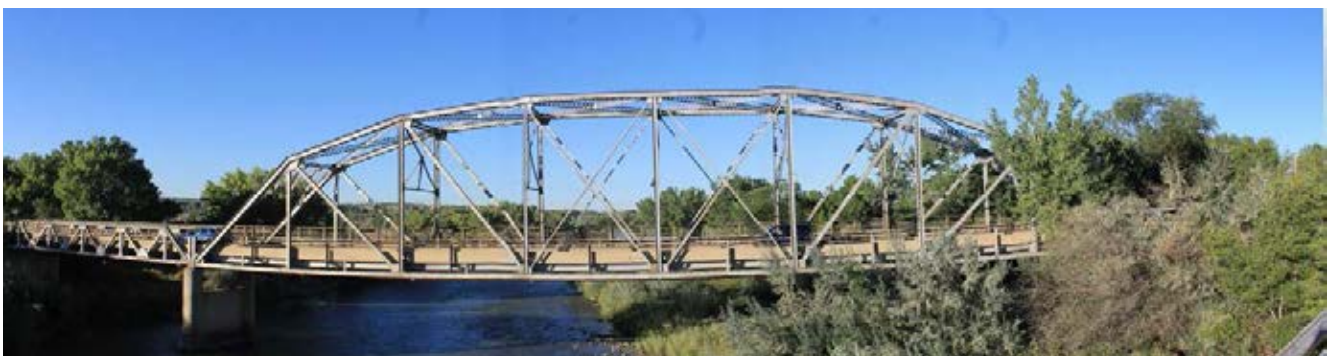
Bridge over the Animas River.
