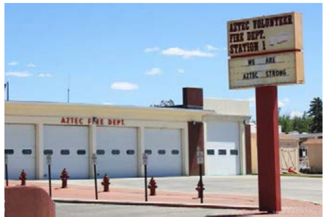
Aztec Fire Department Station 1.
