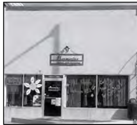
102 N. Main Street - Uptegrove Building
