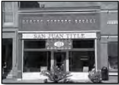
103 S. Main Avenue Waring-Hubbard Building, N&SHR
