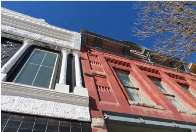
Examples of intricate brickwork in the Italianate and Neo-Classical styles.
