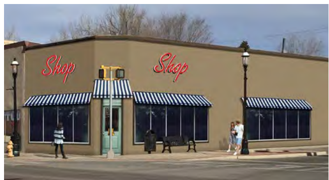
Top: "Ramsey Realty building at Chaco Street and Main Avenue. Bottom: A facade makeover with awnings, new stucco, new windows, new door, and removal of the applied rock surface.
