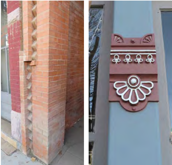
S. Main Avenue buildings exhibit a variety of materials. Left: “zippered brick work; Right: floral motif incorporated into pilaster.
