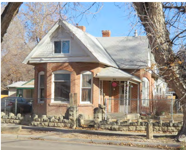
Top: J.M. Randall building, c. 1907; Bottom: single family historic home.
