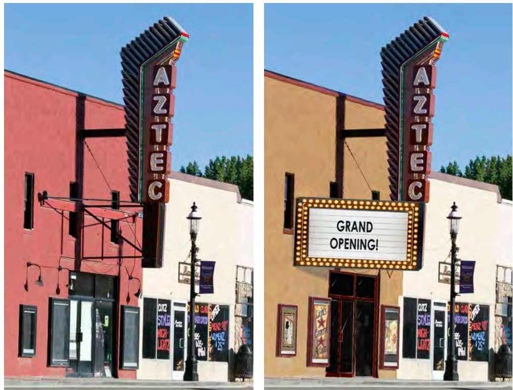
Left: Aztec Theater now; Right: Aztec Theater with a restored sign and marquee and facade improvements.
