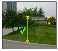
Area identified with the green check mark is the correct calculation for sign height (courtesy of the Signage Foundation).
