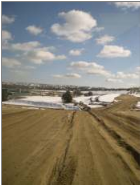
Early grading on Phase 1a of the East Aztec Arterial
