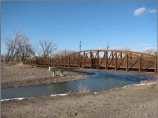
South Animas Pedestrian Bridge
