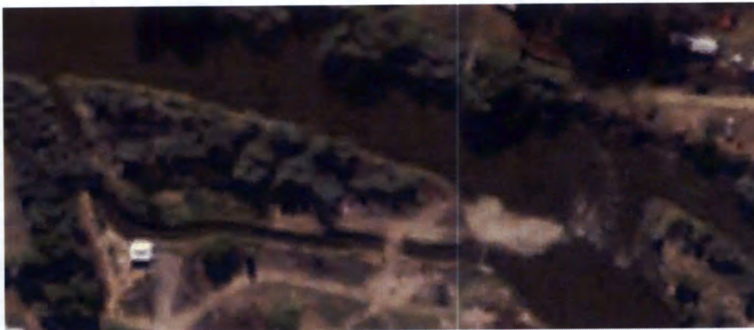
Figure 3: River Diversion with Berm
