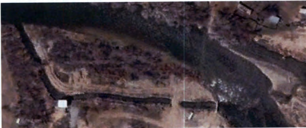
Figure 4: River Diversion without Berm (Eroded)
