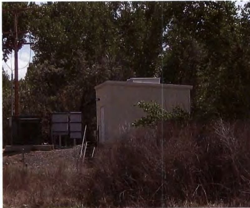
Figure 8: Pump Station (House)
