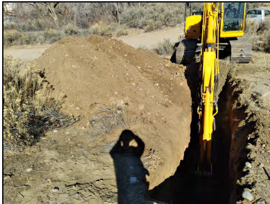
Test Pit Excavation (w/ spoils pile) View Towards the North
