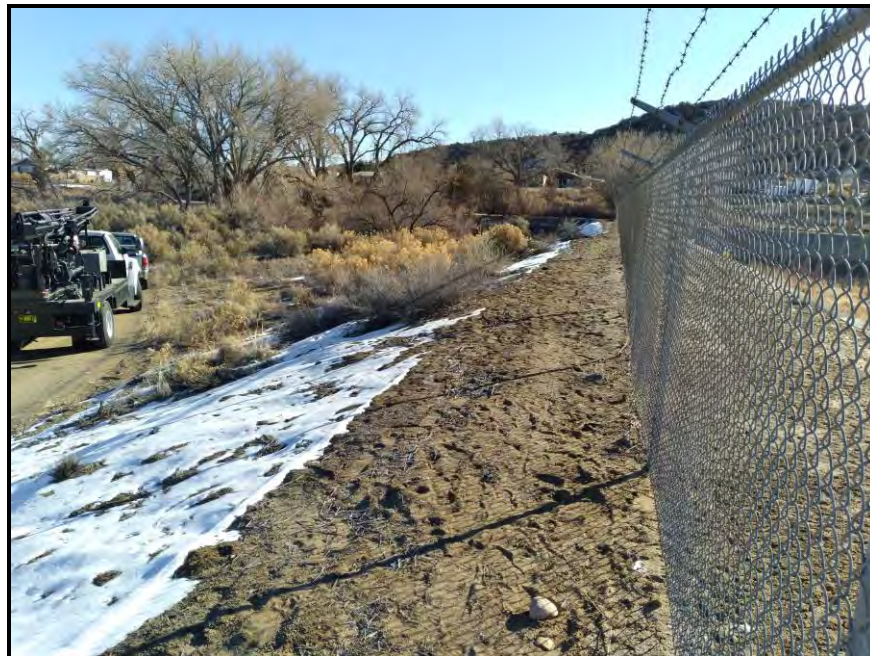
Drill Rig near Boring B-1 View Towards the East
