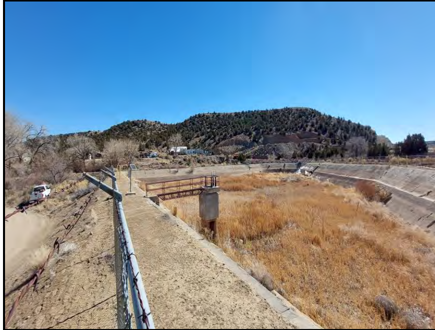
Existing Reservoir and Tower (within reservoir) View Towards the East
