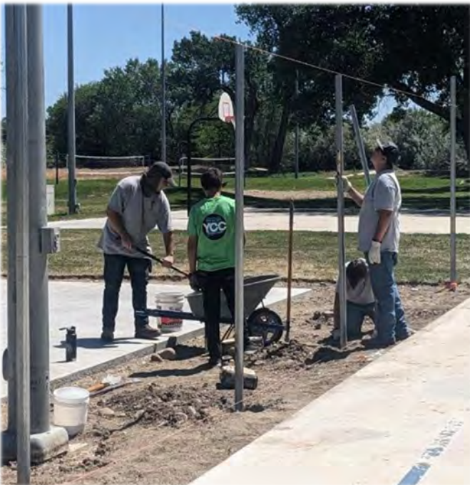
Project 2. Fencing around pickleball court.
