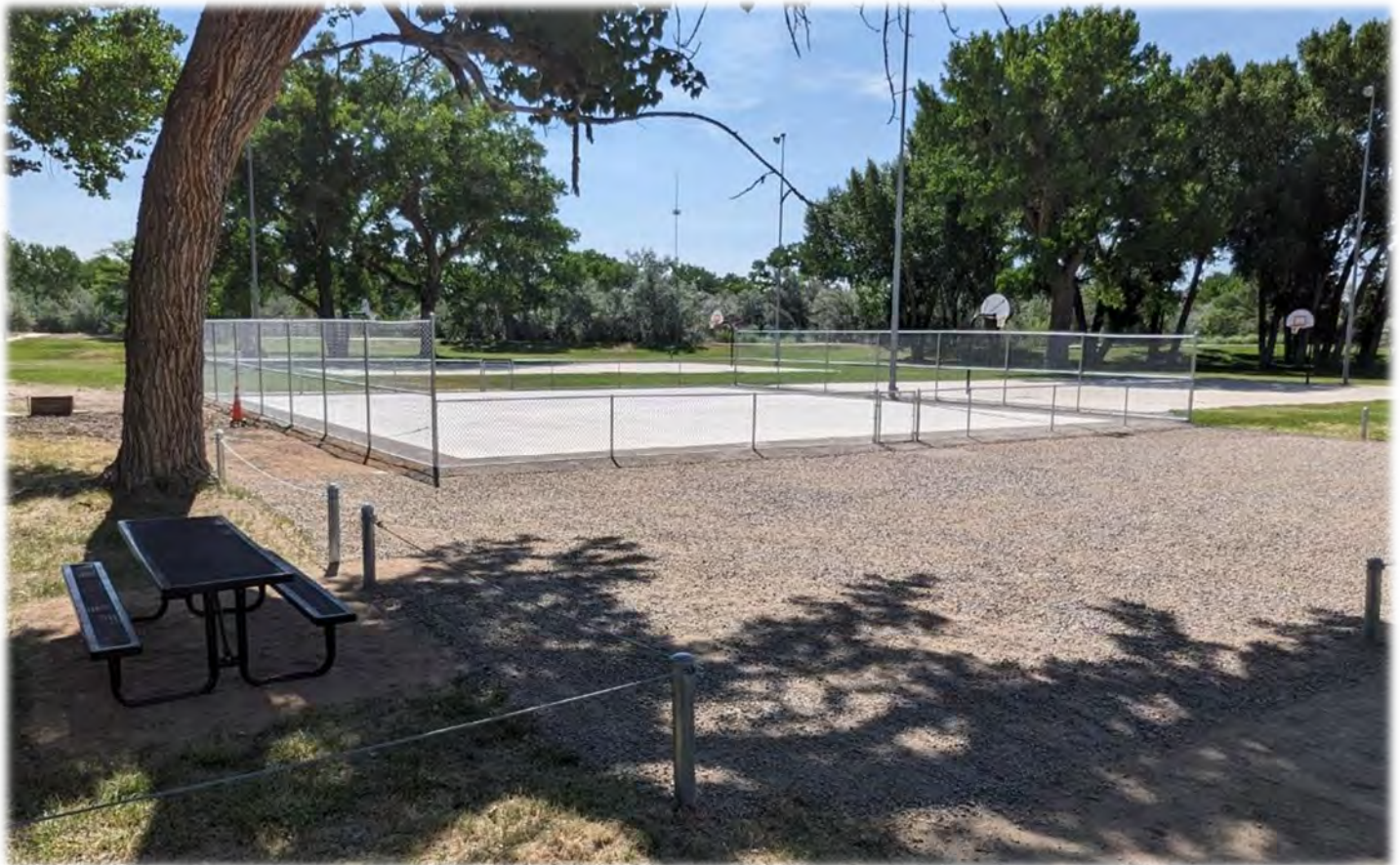
Project 2 & 3. Fencing, landscaping, and parking area completed for pickleball courts.
