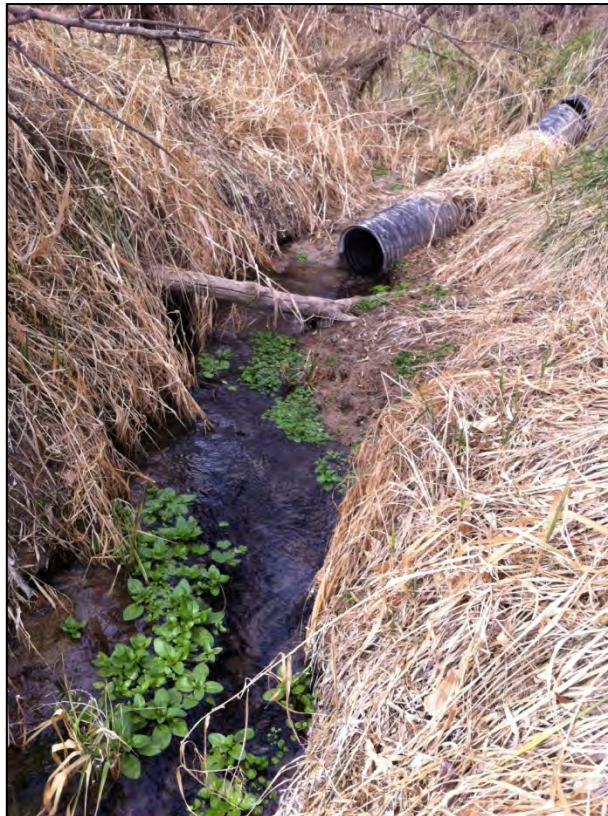
Figure 2. Outfall #2, located in the Harper Valley Subdivision in Farmington, New Mexico.
