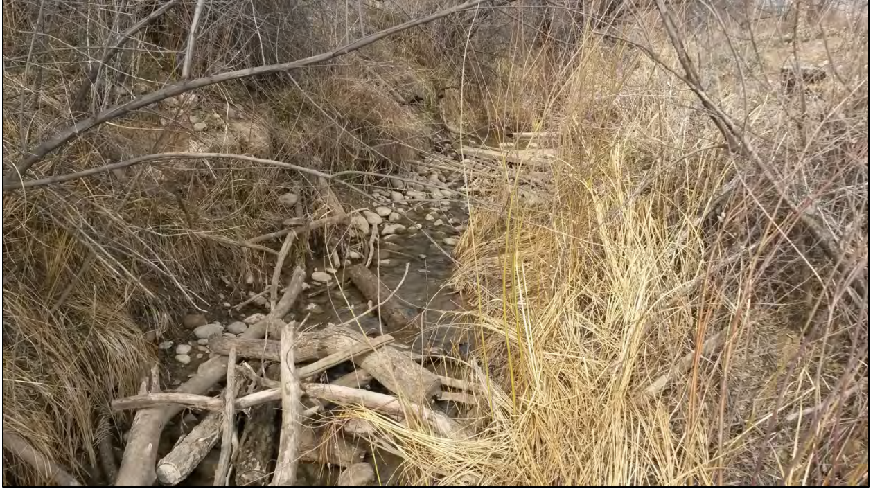
Figure 7. Outfall #10, a channel which discharges to the Animas River at Riverside Park, Aztec, New Mexico.
