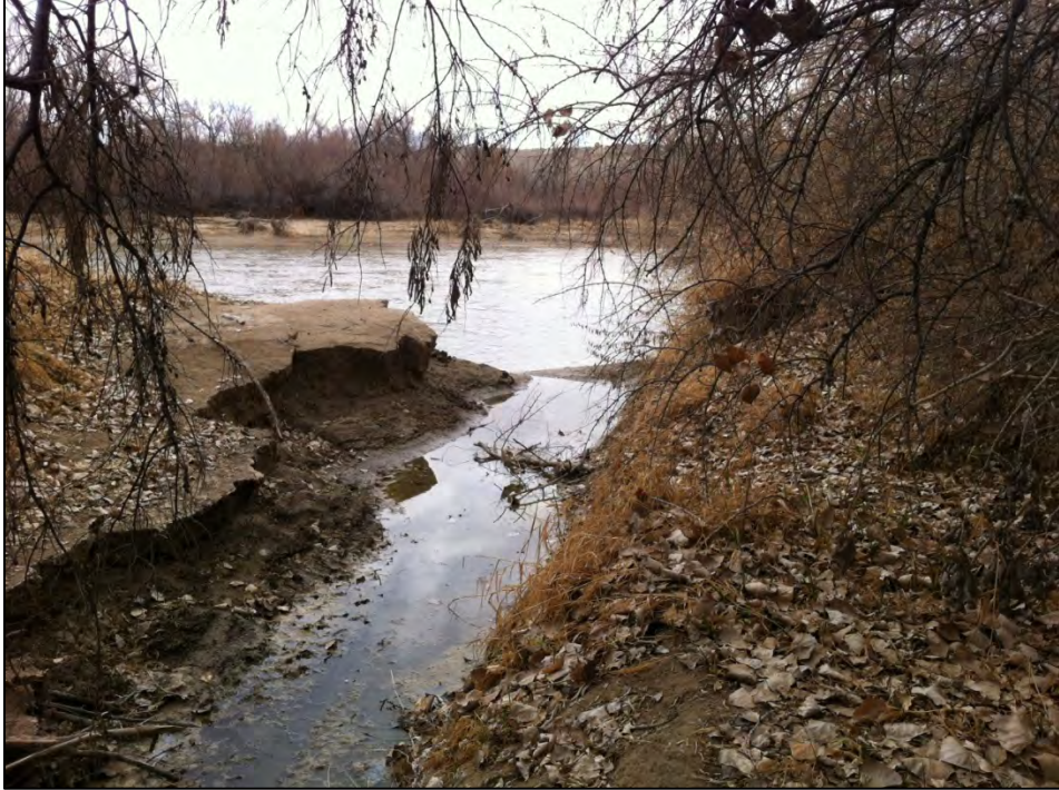
Figure 3. Outfall #3, an open channel fed by an arroyo on the north side of the San Juan River.
