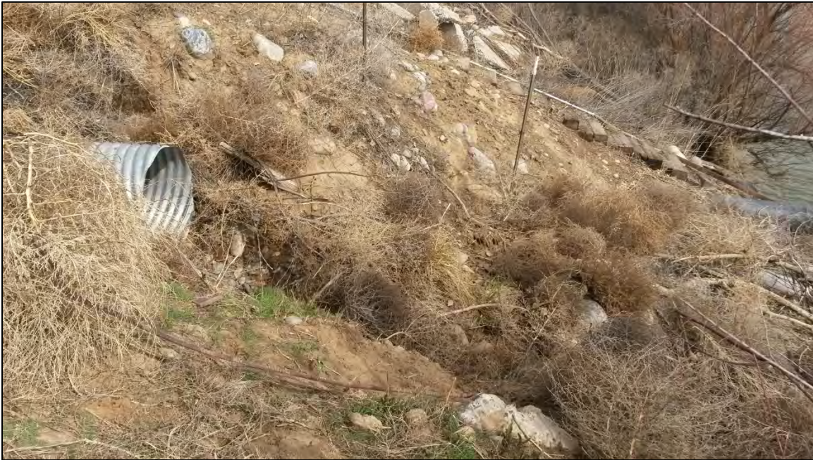
Figure 6. Outfall #9, located at the Animas River near the Aztec Waste Water Treatment Plant.
